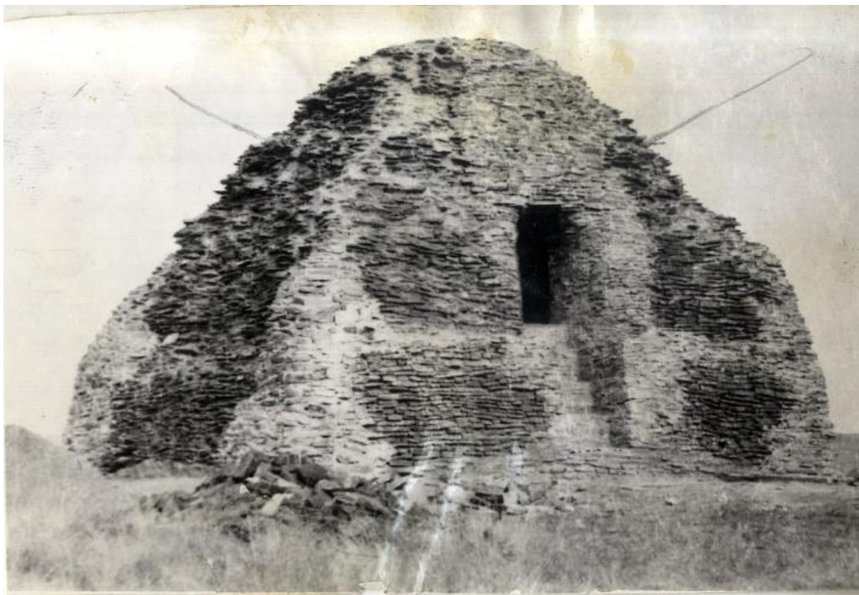
Fig. 1. Historical photo before restoration
