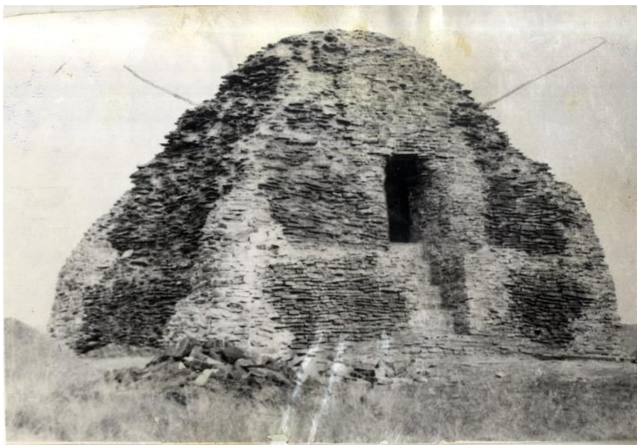
Fig. 1. Historical photo before restoration
